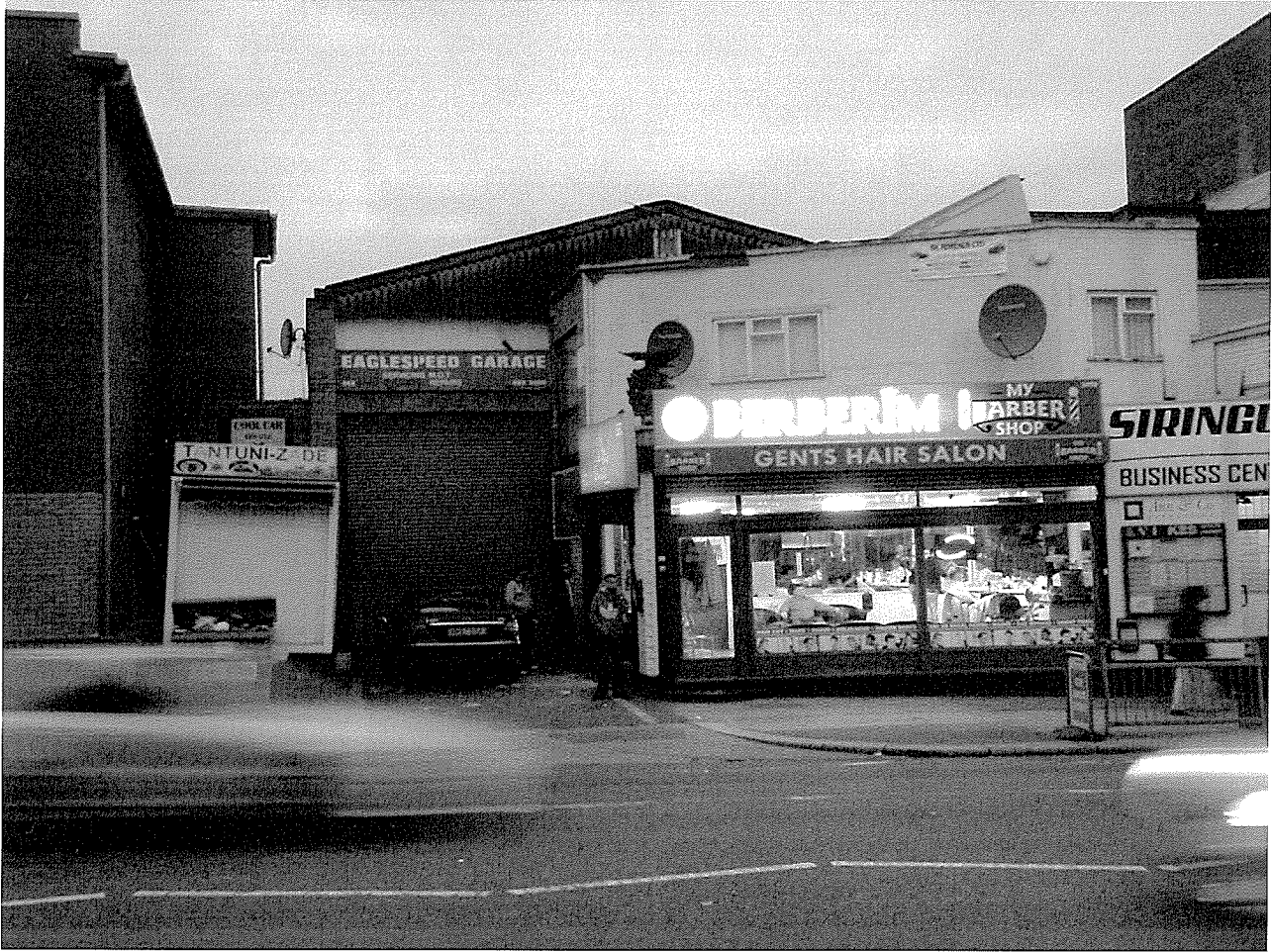
Front of premises
